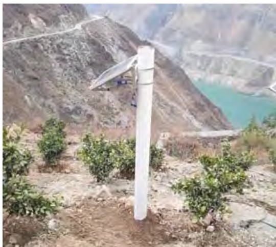
Disaster monitoring system layout site
